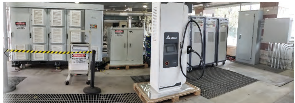
Figure 4: 400kW XFC (SST, Charger Power Cabinet, Dispenser, and DCE from left to right
