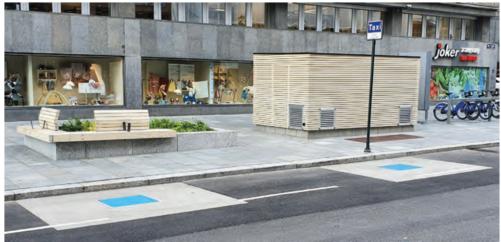
Figure 1: Inductive chargers (blue fields) at taxi stop in Oslo Center. Photo: Erik Figenbaum
