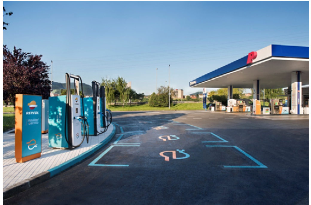
Figure 6: Ugaldebieta (Vasque Country, Spain) ultra-fast recharging infrastructure
