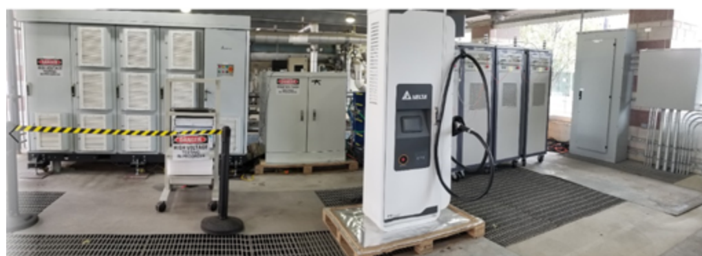
Figure 3: 400kW XFC (SST, Charger Power Cabinet, Dispenser, and DCE from left to right (Source: See Reference [12])
