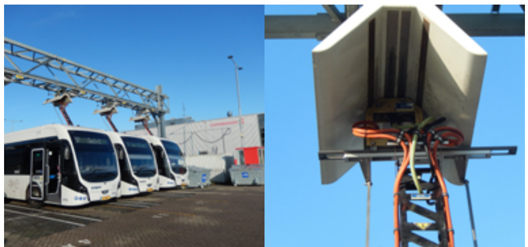
Figure 1: Battery electric buses at charging station in Schiphol Airport
