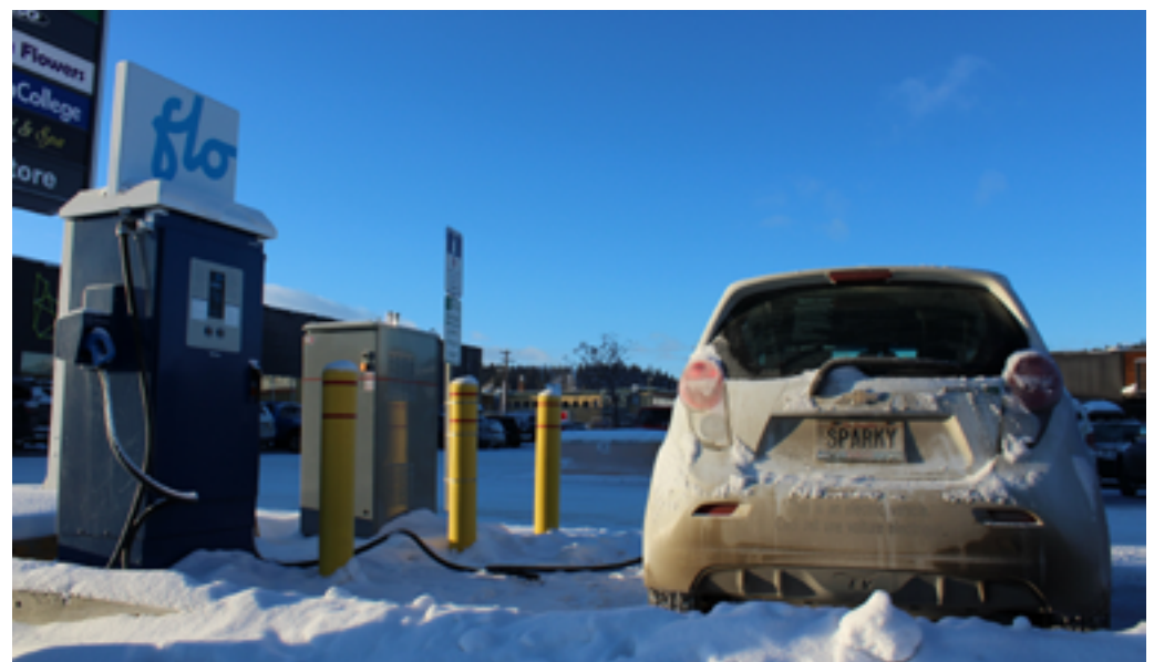
Figure 4: Networked fast charger installed in Whitehorse, YT
