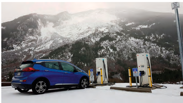
Figure 1: Hope Slide rest area, completed in fall 2018 - two fast chargers, one Level 2 (Source: Government of British Columbia)
