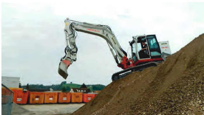
Figure 9: 16 t electric excavator deployed on a building site (Source: www.suncar-hk.com )
