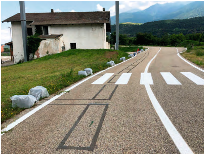
Figure 1: Politecnico Di Torino and FABRIC's on-road WPT installation, Susa, Italy (Source: private)
