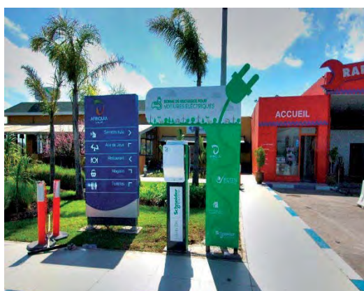
Figure 2: The first charging station implemented within the Green Miles Project, in Afrikaia Settat near Casablanca. The charging station has a power of 22kW (2 x T2S) (Source Iresen)
