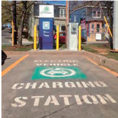
Figure 3: DCFC station in Halifax, owned by NS Power and connected to AddÉnergie's VERnetwork (Image courtesy of AddÉnergie).
