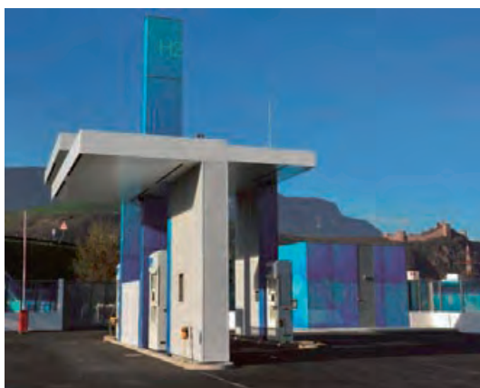
Figure 8: Six 700 bar Hydrogen refueling stations in Bolzano, as part of the CHIC EC project (Image courtesy of CHIC Project)
