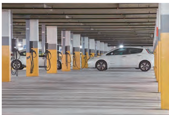
Figure 2: The underground parking at the Bell Campus, in Île des Soeurs (Montréal) consists of 27 Level 2 charging stations installed with support from the 'Branché au travail' provincial government incentive (Image courtesy of AddÉnergie)
