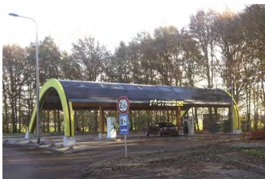
Figure 4: Fastned charging location along Dutch highway (Fastned)
