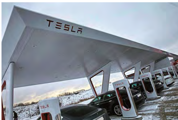
Figure 2: Europe's largest Tesla Supercharger facility in Køge south of Copenhagen (Image courtesy of Tesla)
