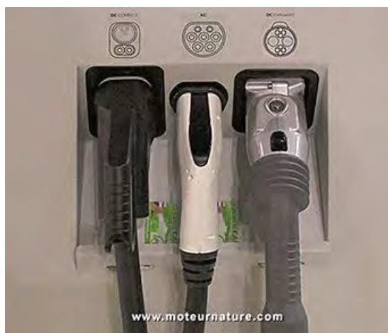
Figure 3: DC combo2, AC, and DC CHAdeMO plugs at a charging station (Image courtesy of www.moteurnature.com )
