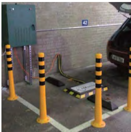
Figure 1: An induction charger – ESB Head Office
