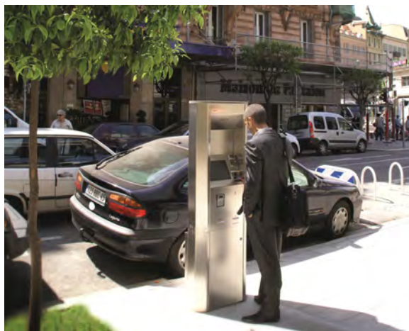
Fig. 19.1 Enstos Chago kiosk in Nice. (Source: Enstos [ http://www.ensto.com/newsroom/references/evcharging/101/0/spot_ensto_chago_kiosks_along_garibaldi_2 ])
