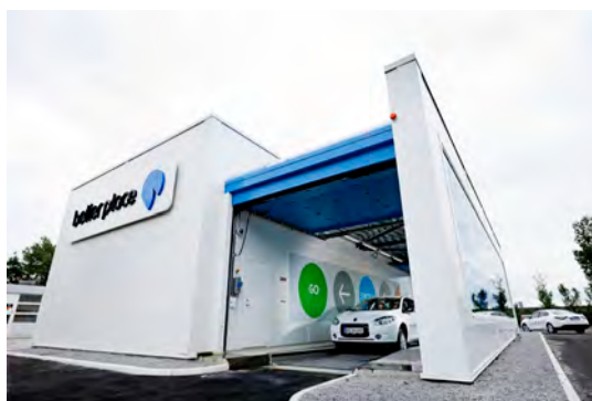
Fig. 16.3 The first Danish battery switch station in Gladsaxe north of Copenhagen. (Photo courtesy of Better Place Denmark.)
