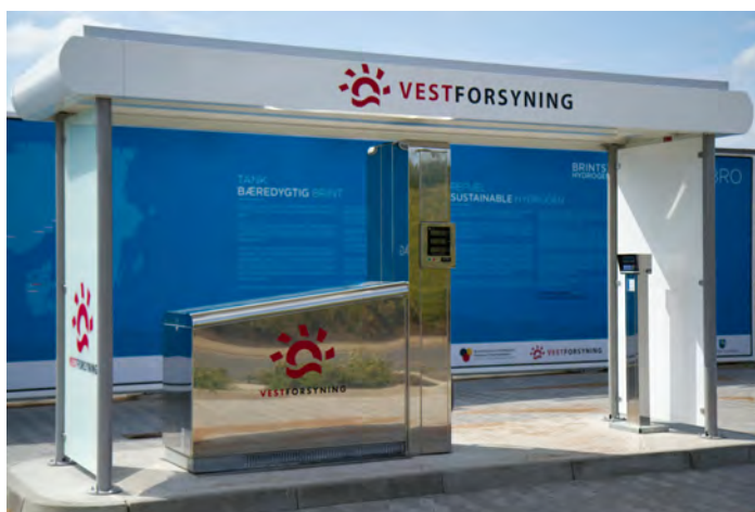
Fig. 16.1 The 700-bar hydrogen station in Holstebro, Denmark enables refueling in 3 minutes. (Photo courtesy of H2 Logic.)
