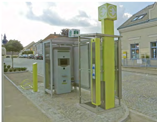
Fig. 14.6 Charging point from an adapted phone booth in Maria Taferl (Lower Austria) (Source: Everynear).
