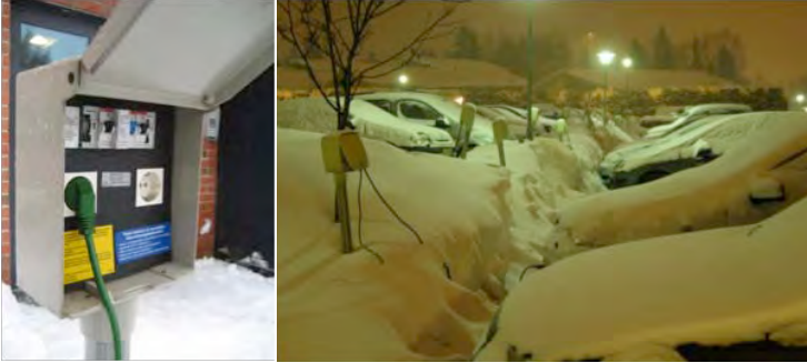
Fig. 19.4 “Block heater pole” and a view from a car park of a row house condominium. There are typically standard “2-hour” timers at block heater poles. The starting time is selected by the user, but the heating time is fixed for two hours from the start.
