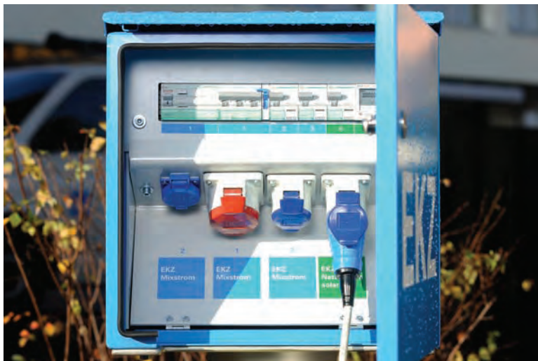
Fig. 27.9 Typical outlets for 16 A (blue) and 32 A (red) using CEE industry plugs and sockets. (Photo courtesy of EKZ.)
