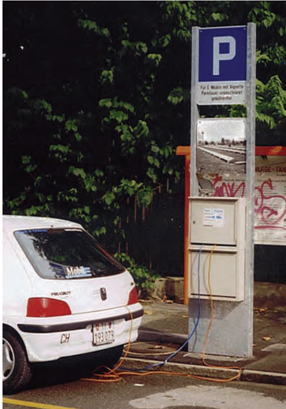
Fig. 27.8 Park & charge facility at the railway station in Thun. (Photo: Solarcenter Muntwyle)
