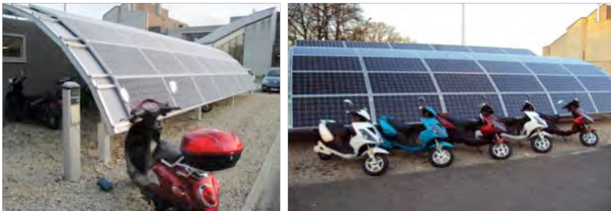
Fig. 15.4 “Green” Charging Station for electric scooters. (Photo courtesy of KHLim.)
