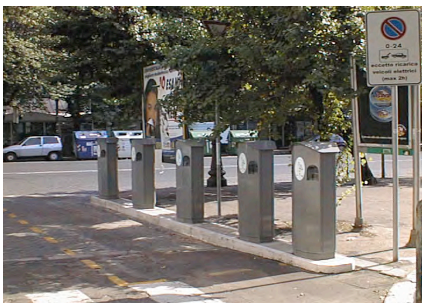
Fig. 7.3 Public charging stations for electric scooters in the city of Rome, Italy. (Photo: Fabiana Marconi.)
